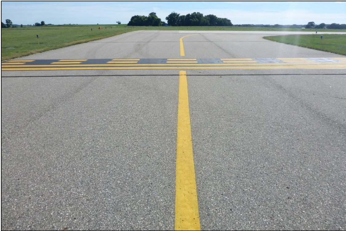
12Y CTB 001 (PCI = 88) Photo taken pre-maintenance (crack seal and slurry seal)
