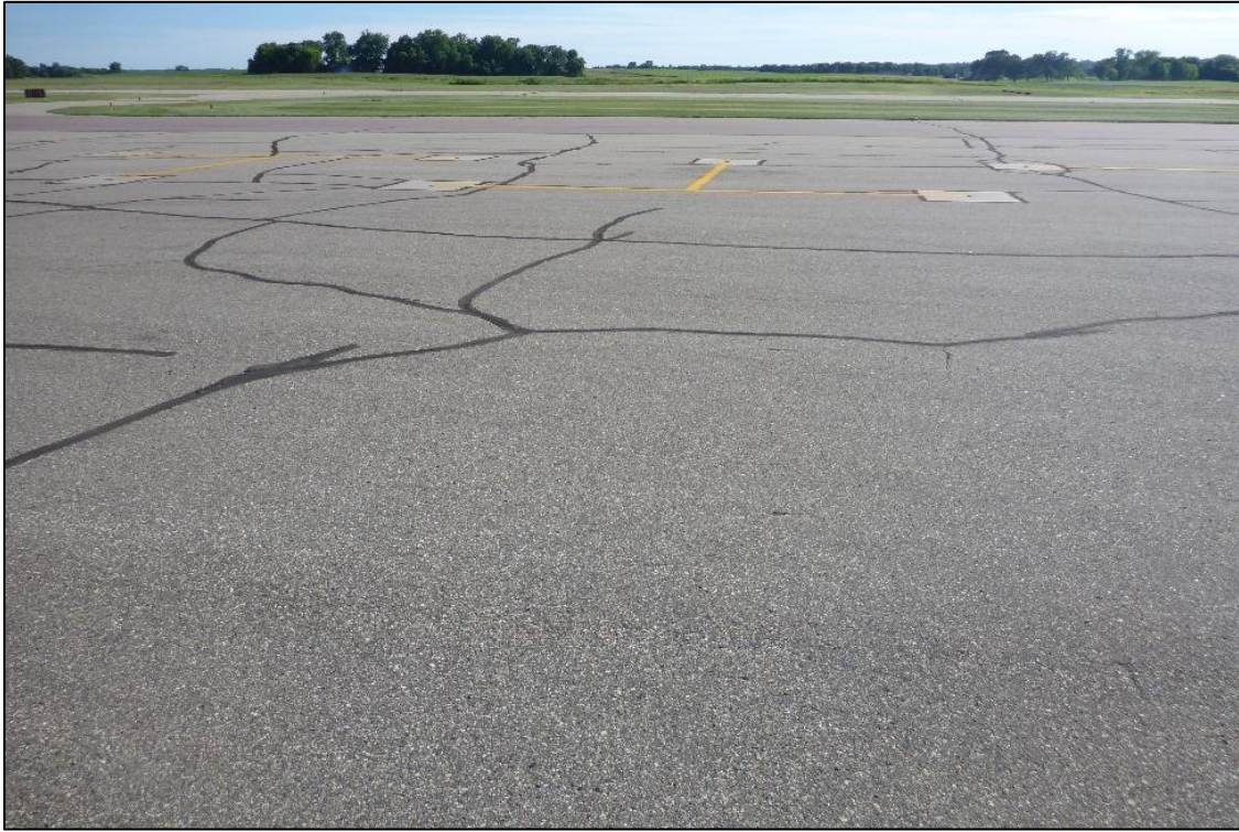
12Y APA 001 (PCI = 72) Photo taken pre-maintenance (crack seal and slurry seal)
