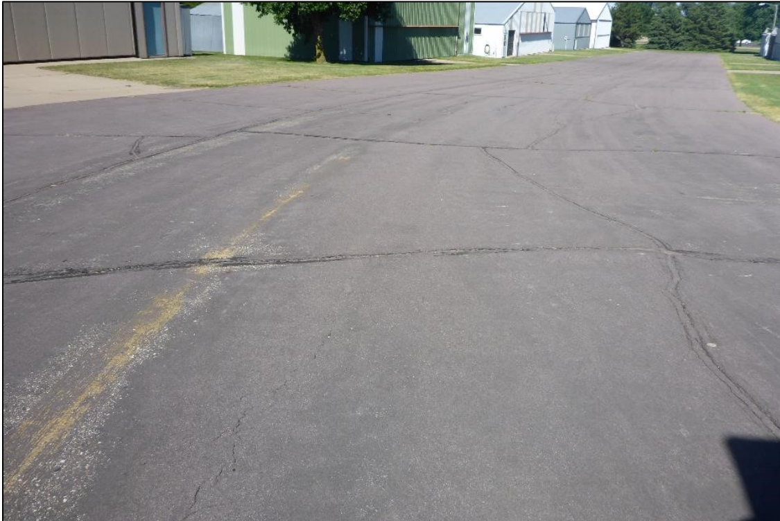
12Y TLC 001 (PCI = 66) Photo taken pre-maintenance (crack seal and slurry seal)
